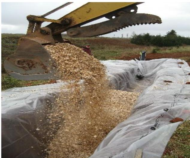
The Darnley Bio-Filter is a pit lined with plastic, the same heavy plastic used as a vapour barrier in home construction, and then filled with wood chips. The water from the tile drain enters the pit, and microbial activity in the pit removes 50 to 80 % of the nitrates in the water. The pit can remain functional for 20 years or more.
